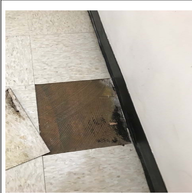
Trailer #20 Below the 1 st window from the entrance
