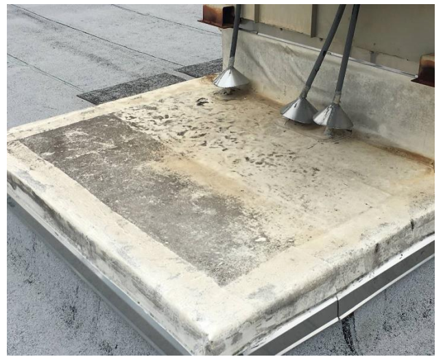
Photo 6: Suspected mold growth on HVAC machine base area
