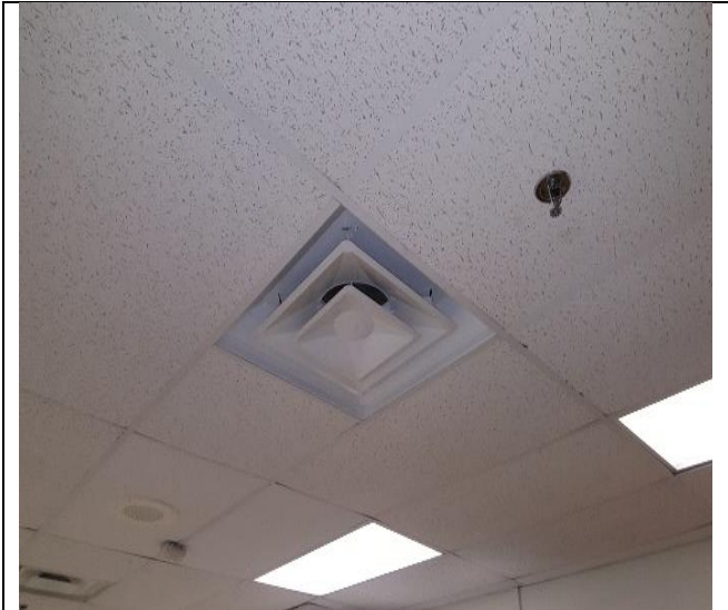
Photo 1: AC diffuser from inside a room
