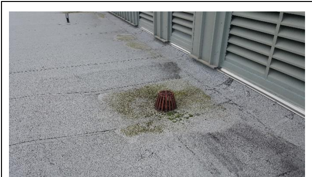
Photo 13: Suspected mold growth on the roof
