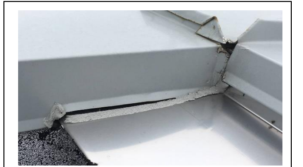
Photo 16: Representative location for roof flashing joint cracks
