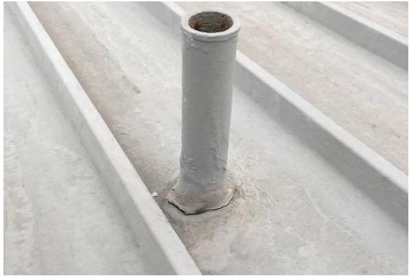
Photo 17: Cracked sealant at the roof penetration point area
