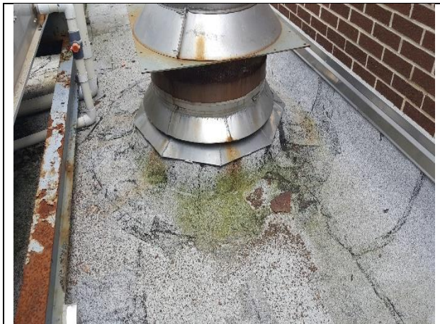
Photo 11: Suspected mold growth on the roof
