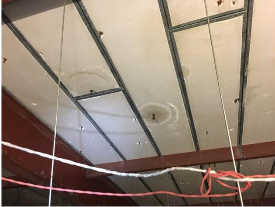
Photo 18: Roof penetration point where signs of water intrusion
