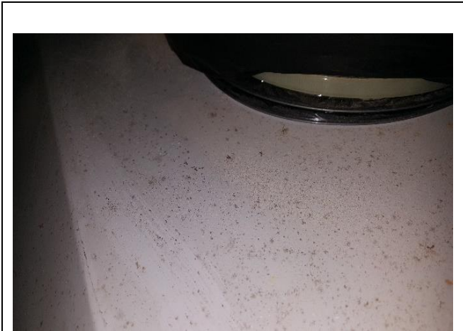
Photo 3: Suspected mold growth on AC diffuser
