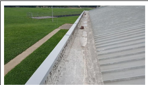
Photo 14: Suspected mold growth on angle roof landing area
