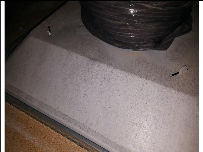
Photo 2: AC diffuser from above the ceiling
