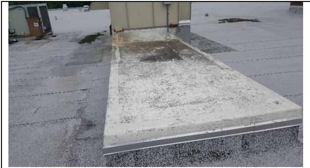
Photo 15: Suspected mold growth on HVAC machine base area
