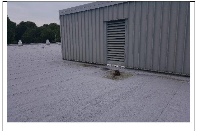
Photo 12: Suspected mold growth on the roof
